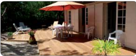
Garden spaces: cladding and decking
