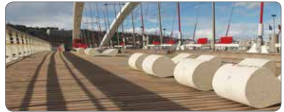
Public Spaces: Bridge and Boardwalk Decking
